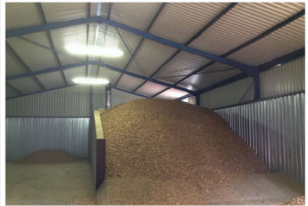
immediate fuel store filled with woodchip
