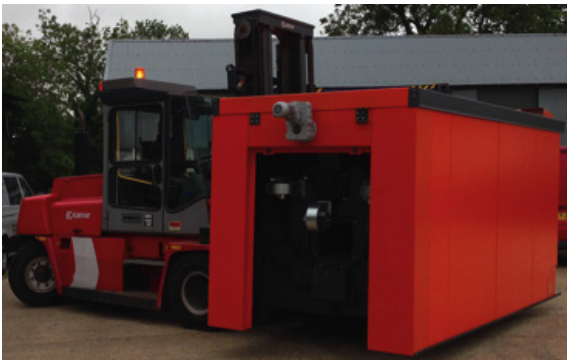
Heizomat RHK AK 500kW boiler being manoeuvred into position for containerisation
