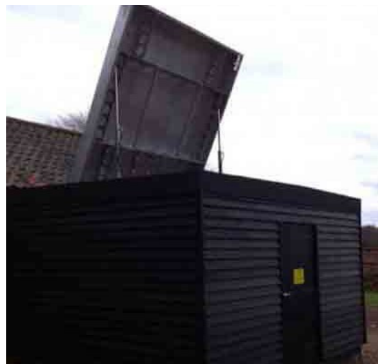
Hydraulic lid fuel store designed and constructed by Nexus Energy
