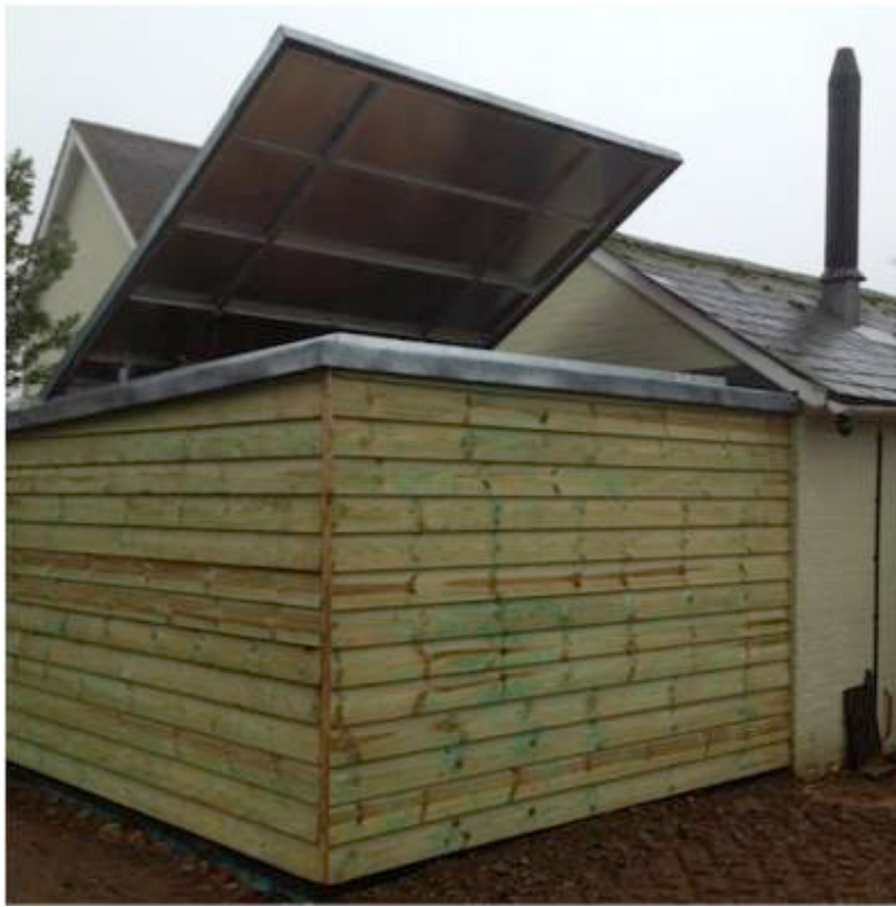
Nexus Energy–Custom designed and constructed hydraulic lid fuel store.
