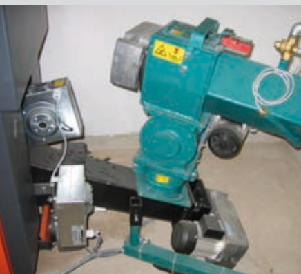
4 chamber rotary valve with counter blade.
