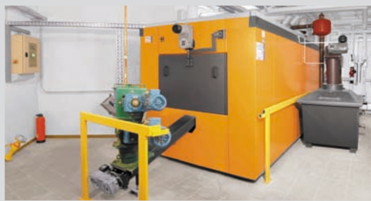
Our RHK-AK boiler type is available with a output range of 30-990 kW.
