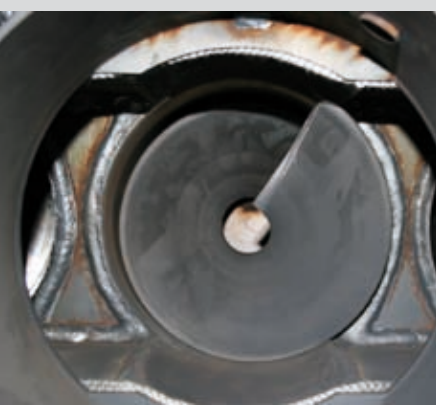
De-ashing augers for cleaning the heat exchanger.
